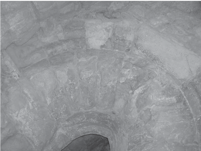
Fig. 30: Limassol Castle, vestibule between lower level of cells and réduit , detail of fire-damaged masonry on the upper part of thirteenth-century Gothic clerestory window [M. Olympios].
